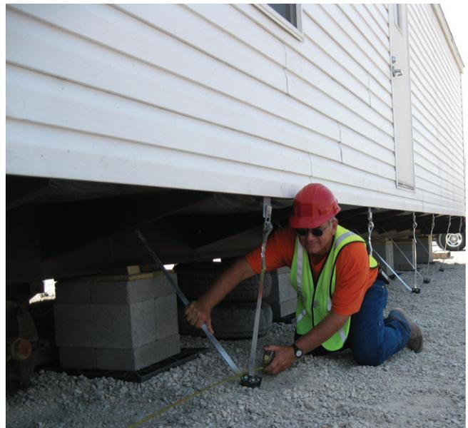
*Ronnie Mann, a PSC Manufactured Housing Field Inspector, inspects the installation of the anchors under a FEMA Home at the Joplin Airport Site.*
